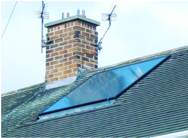
Above - A 2.75m 2 meter Zen flat plate collector mounted 'in roof' with flashings.
