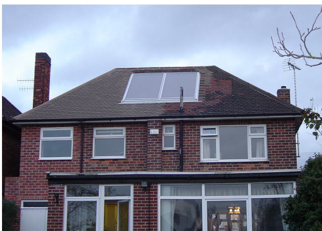
Above - A 5.4m 2 Schuco 'in roof' collector flashed into a roof. (Installed by T4).
