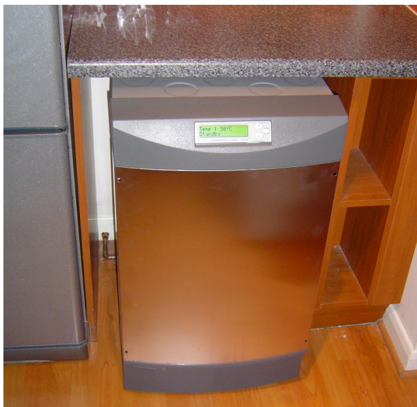
Left and above - The Whisper Gen co-generation system, about the size of a dish washer, up to 1.2kW electrical, and 8kW thermal output. An oil fuelled version of this boiler is available.
