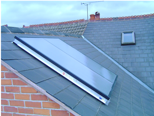
Below - the same type of panel installed 'on roof'. (Both drain back installs by T4).
