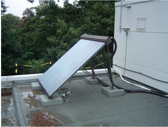
Above - Evacuated tube collector mounted on a flat roof.
