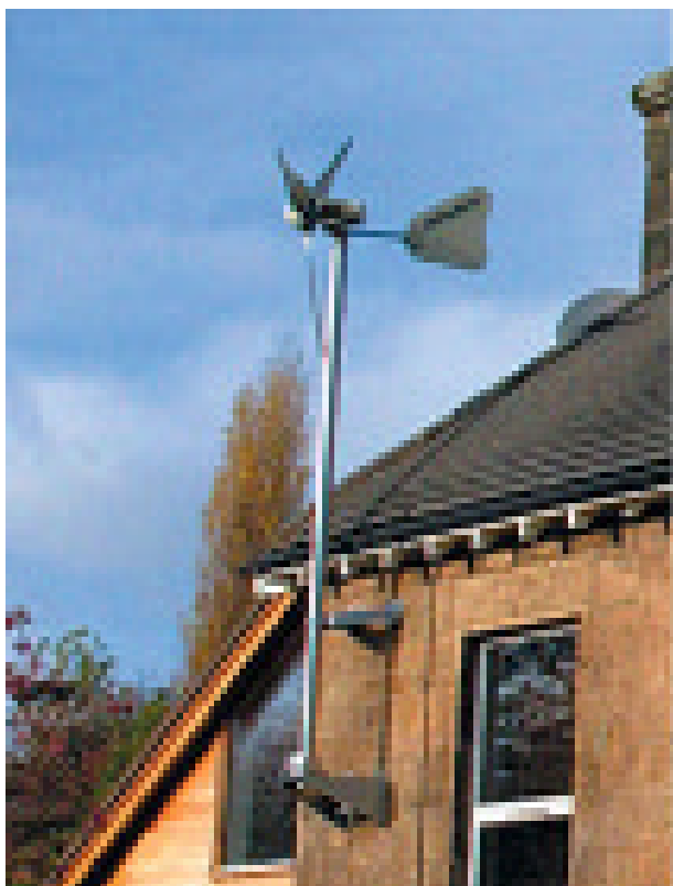
Left - A Windsave turbine. 1kW nominal power output at a 12.5 \text{ ms}^{-1} wind speed.
