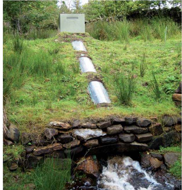
Figure 2.8 A buried 1 kW screw at Bonfield Ghyll, North York Moors National Park, minimising landscape impact (photo courtesy of MannPower)
