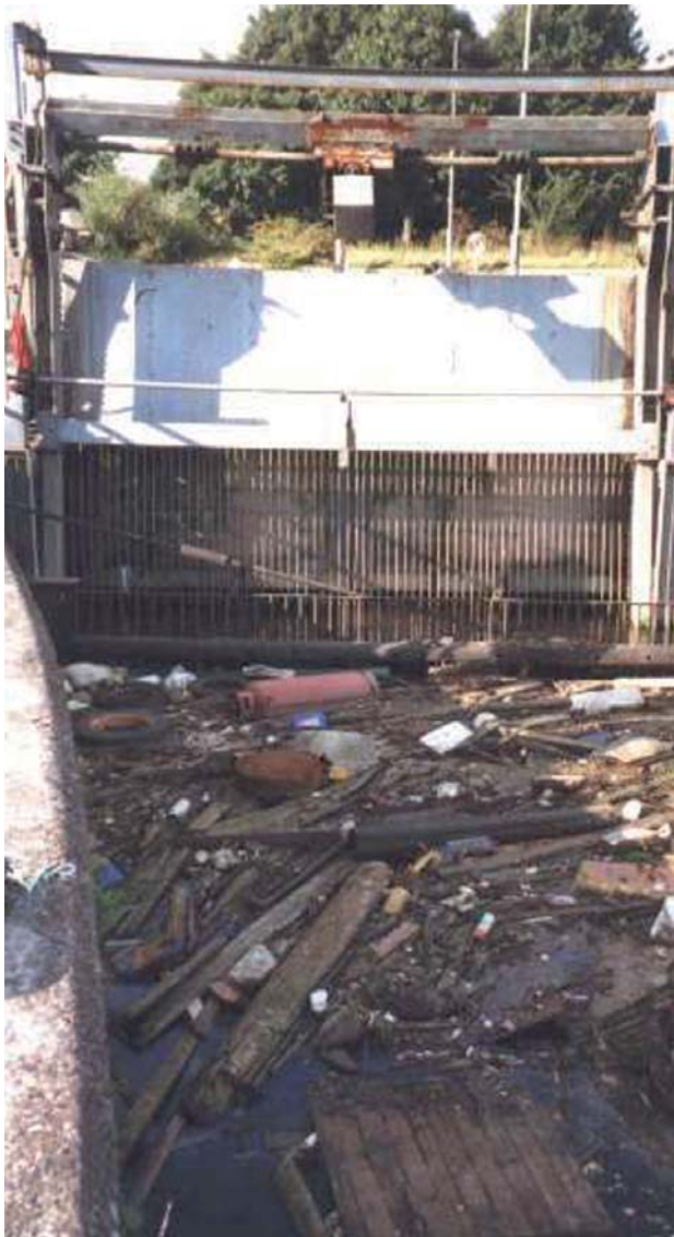
Figure 2.14 Mechanically raked bar screen at Barton, near Manchester, showing build up of debris (photo courtesy O. Paish)
