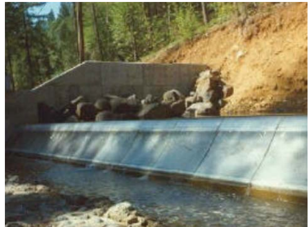
Figure 2.17 A Coanda or 'wedge-wire' screen (courtesy of BHA)
