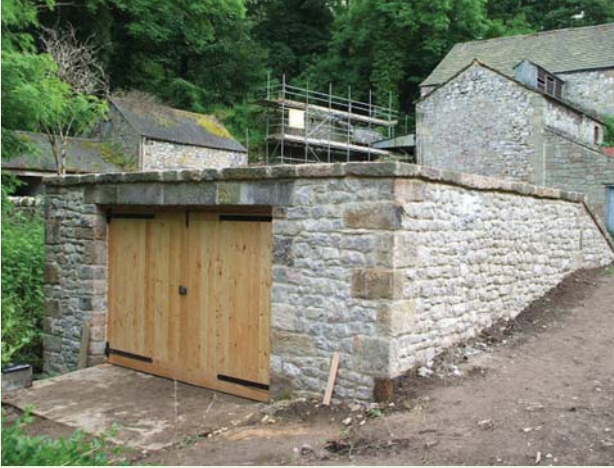
Figure 3.2 The new turbine house at Alport Mill faced with local stone (photo courtesy of Derwent Hydro)
