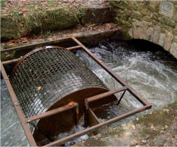
Figure 2.15 Self-cleaning drum scheme at the Old Walls scheme, Dartmoor
