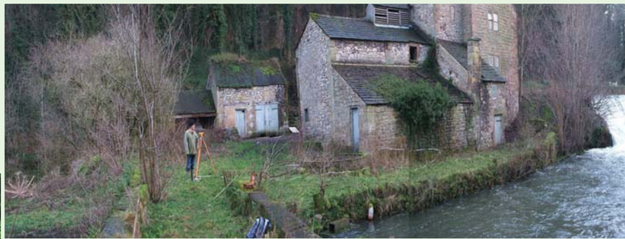
Figure 3.3a/b Before and after pictures of the Alport Mill scheme showing the buried powerhouse at left (photos courtesy of Derwent Hydro)
