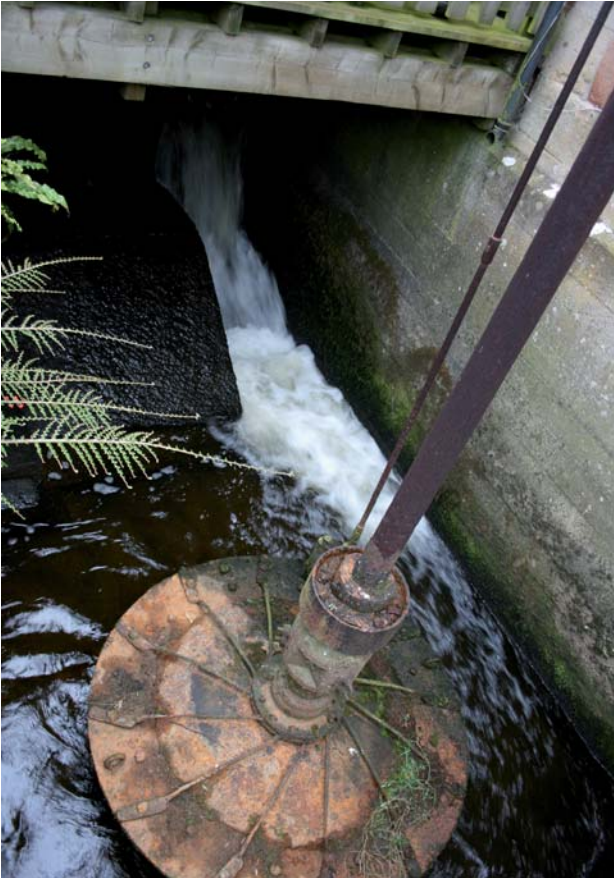
Figure 5.3 The original turbine in situ at Hodgkinson's Mill in Baslow
