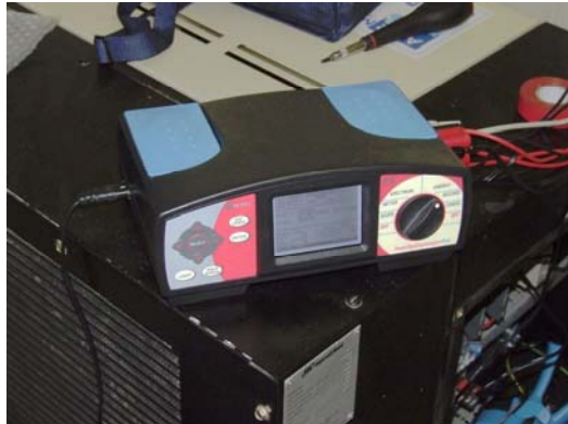
Left, electrical data logging for one of Central Joinery's compressors
