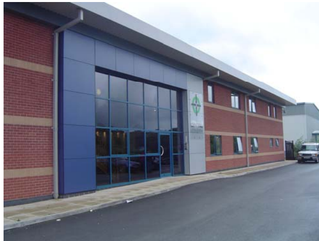
Left, Central Joinery factory and offices, recently constructed in a purpose-built unit
